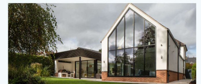
IDS Glass Curtain Walling | RAL 9011 Graphite Black Curtain walling including angled fixed frames
